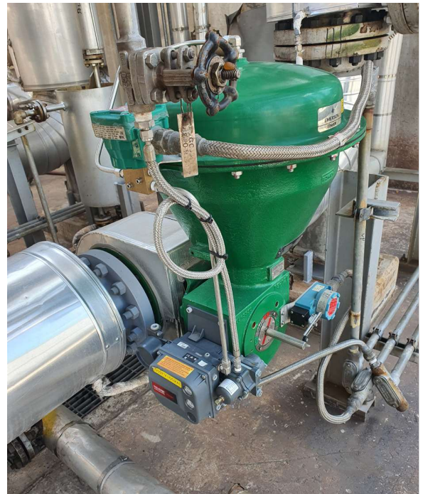
Fisher Vee-Ball Cavitrol™ Hex Trim combines the advantages of Vee-Ball capacity and rangeability with Cavitrol Hex Trim that helps prevents cavitation.
