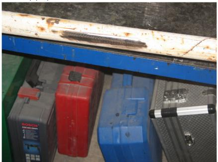
Now the pipe is ready and the clamp-on sensors could be installed.
