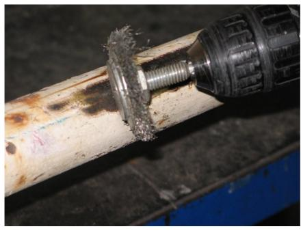
4. The pipe portion in which the sensor will be mounted should be completely clean:
