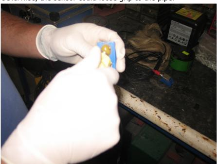
9. Now sensors could be installed by using a fixing bracket:
